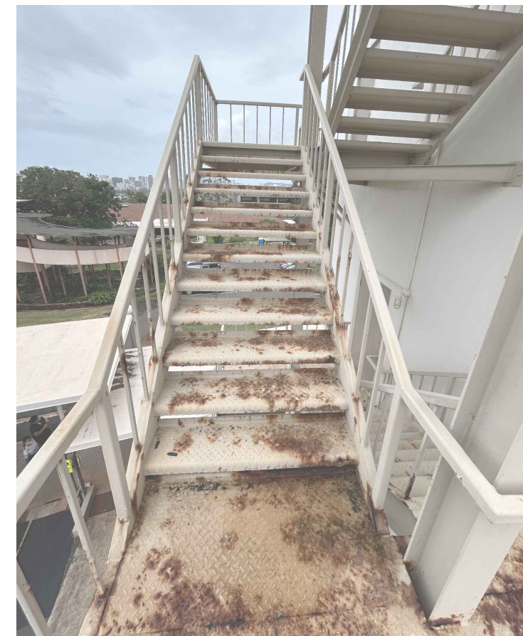
F FIRE ESCAPE 2 - SECOND FLOOR
