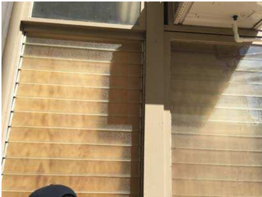
Photo #11: Administration building. Windows with asbestos containing caulking.
