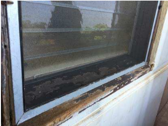
Photo #15: Trotter building. Wood windows with non-asbestos containing caulking.
