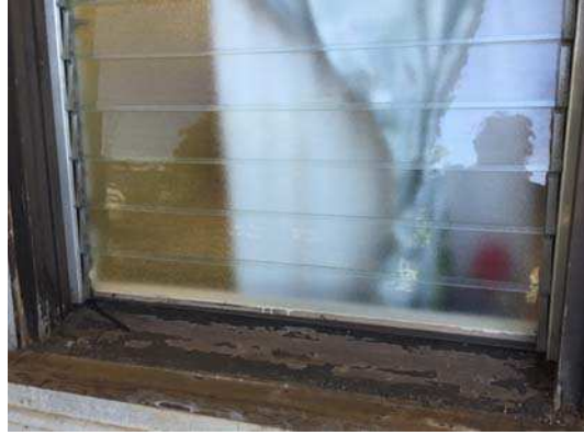
Photo #14: Trotter building. Wood windows with non-asbestos containing caulking.
