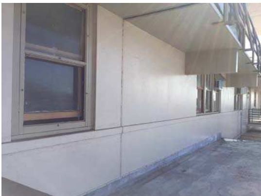
Photo #5: Young building. Wood windows with asbestos containing caulking.
