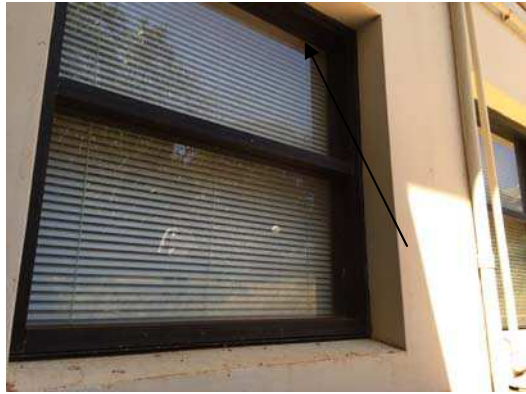
Photo #16: Trotter building. Metal windows with non-asbestos containing caulking.
