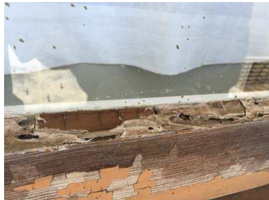
Photo #4: Young building. Wood windows with non-asbestos containing glazing (interior of the frame).
