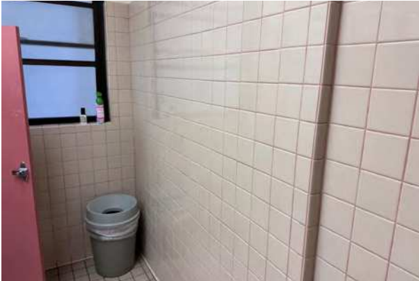
Photo 1P: Ceramic wall tile. Glazed beige coating. Non-LBP, below the laboratory reporting limit.
