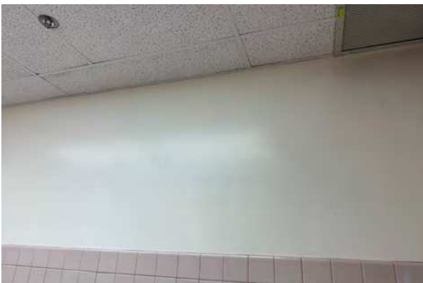
Photo 5P: Concrete wall (upper portion). Beige paint with lead.
