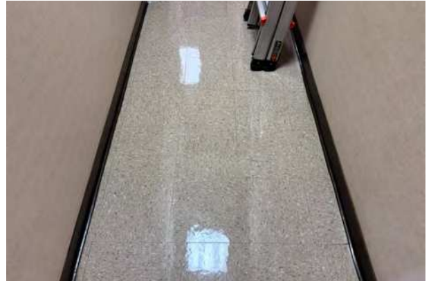
Photo 2: 12"x12" tan vinyl floor tile with black mastic and concrete. Non-ACM.
