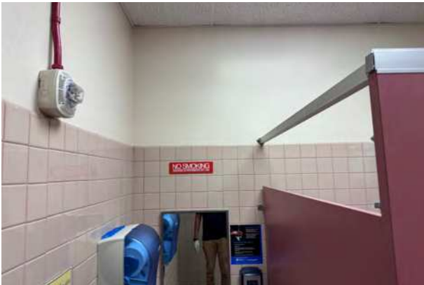
Photo 3P: Drywall partition (upper portion). Beige paint with lead.
