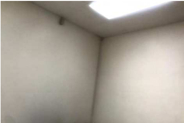
Photo 9: Beige painted white drywall and joint compound. Non-ACM.
