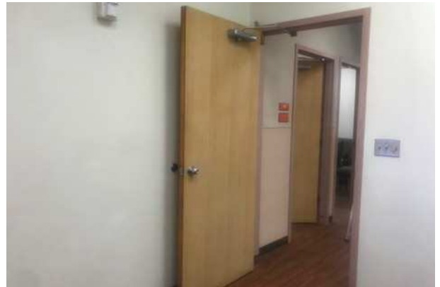
Photo 10: Beige painted brown drywall and joint compound. Non-ACM.
