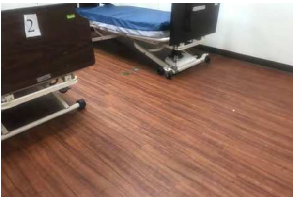
Photo 11: Brown wood design with tan mastic over vinyl floor tile and black mastic/concrete coating. Non-ACM.
