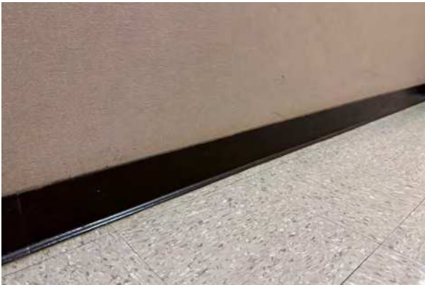
Photo 3: 4" brown vinyl cove base with brown mastic. Non-ACM.
