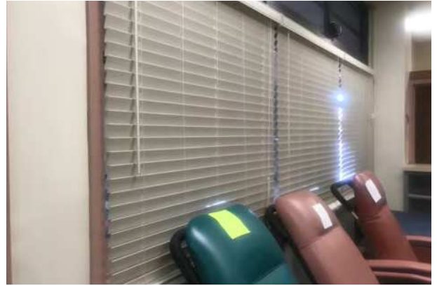
Photo 14: Gray window caulking. Non-ACM.
