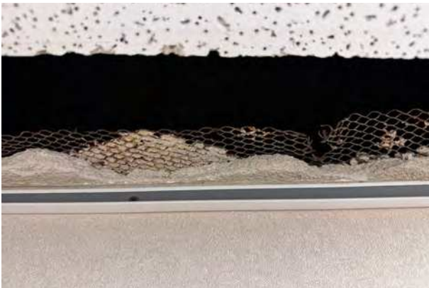
Photo 5: Plaster wall/lath. Non-ACM.
