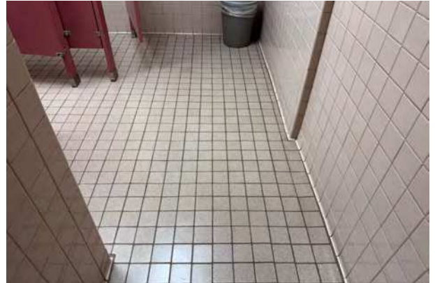
Photo 2P: Ceramic floor tile. Glazed tan coating. Non-LBP, below the laboratory reporting limit.
