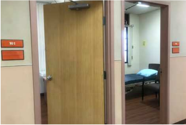
Photo 13: White door caulking. Non-ACM.
