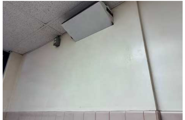
Photo 4P: Plaster wall (upper portion). Beige paint with lead.
